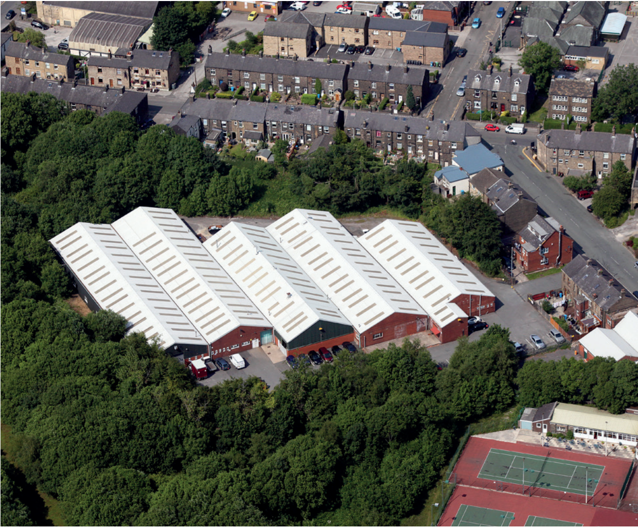
Aerial view of our manufacturing facility near Manchester
