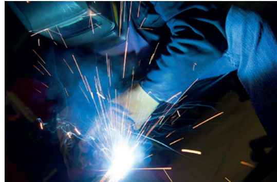
On-Site coded welders
