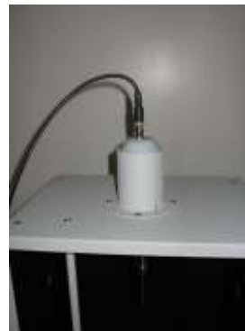
Proper installation of horn
